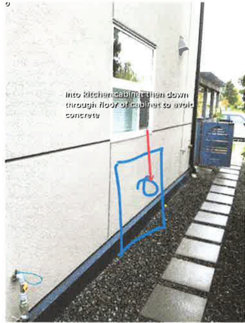
Unit 14 location, using kitchen cabinet for pipe location
