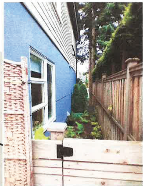
Rear of Unit 6 looking east
