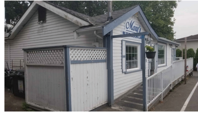
VIEW LOOKING SOUTH EAST - EXISTING RAMP
