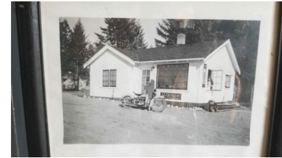
VIEW LOOKING NORTH EAST, HISTORIC PHOTO
