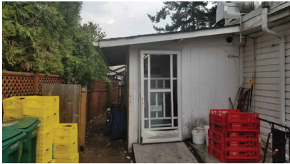
VIEW LOOKING EAST, EXISTING SIDE ENTRY LOADING AREA
