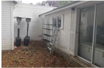
VIEW LOOKING WEST, REAR ALCOVE MAIN STRUCTURE TO THE LEFT OFFICE AND STORAGE TO THE RIGHT
