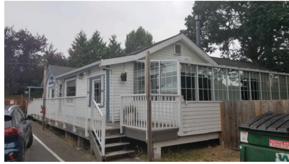
VIEW LOOKING NORTH EAST - FRONT ENTRY STEPS CONSERVATORY
