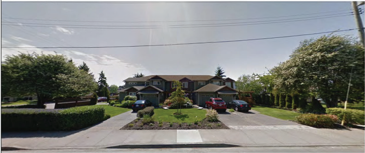
STREETSCAPE: LOOKING SOUTH
