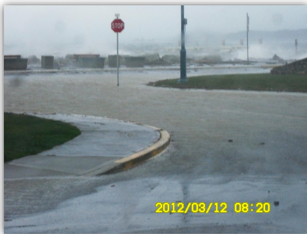
March 2012 Flooding on First Street
