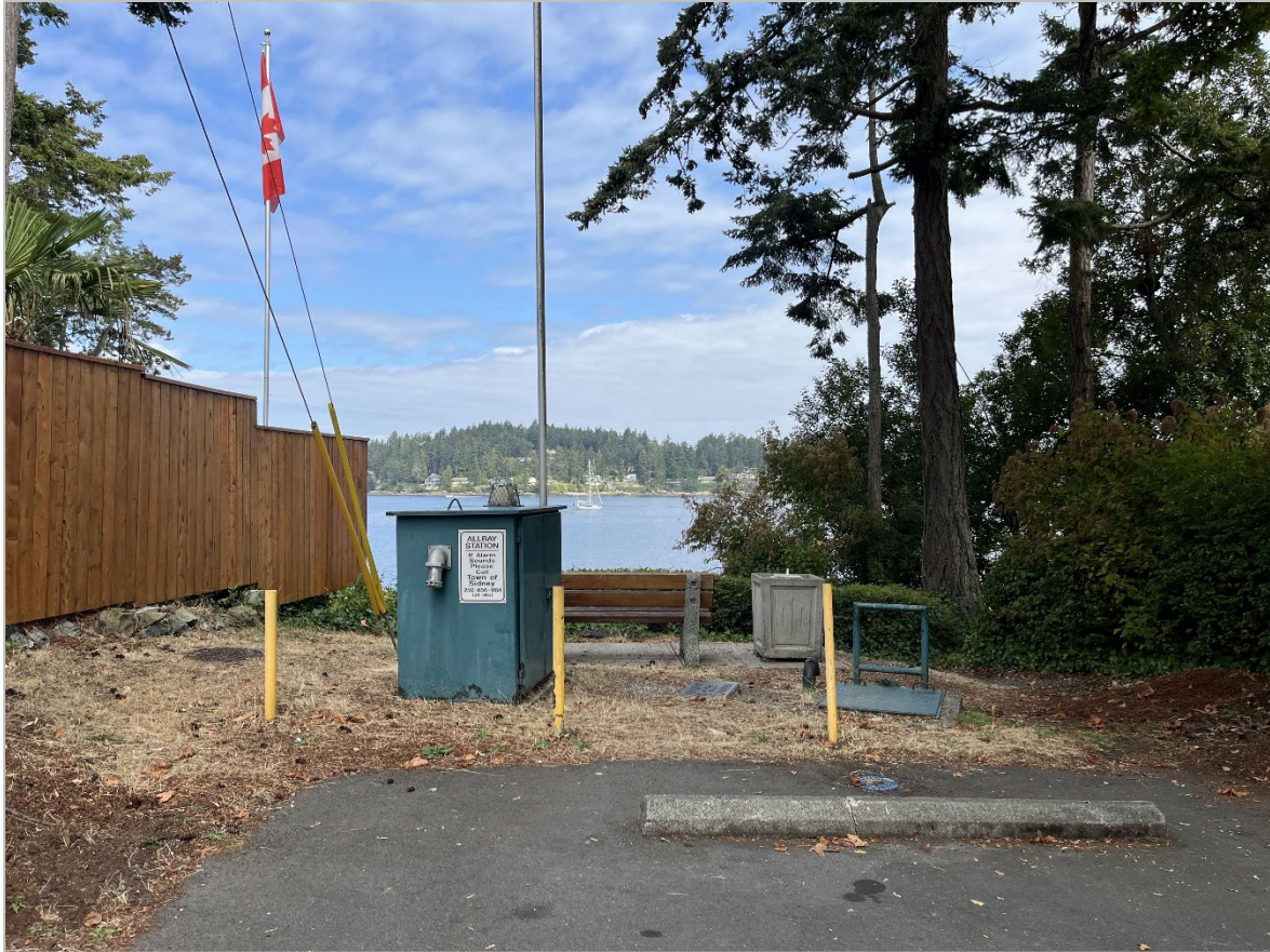
Photo 7. Typical sewer pump station condition and context in Sidney.
