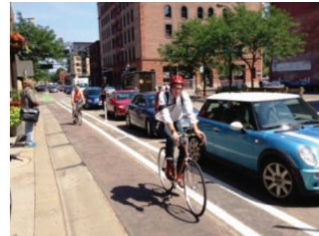
II. PRIORITY BIKEWAY (Fifth Street) On-street cycling facilities that are physically separated from vehicle traffic by buffers, landscaping, or by locating on-street parking between vehicle and bicycle travel lanes.
