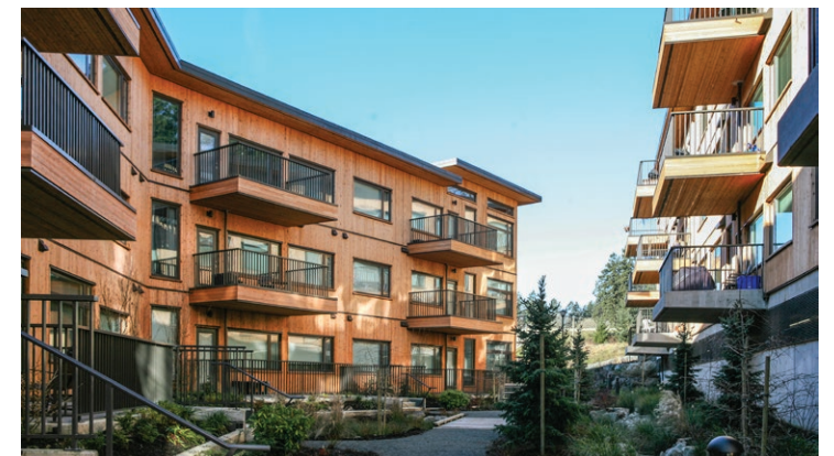
Figure 3b: An example of how building articulation can provide adequate spatial separation between residential units
