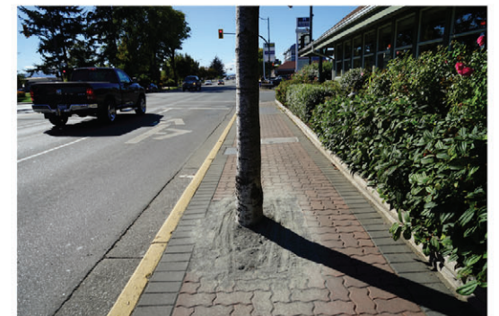
Existing Sidewalk (North Side)
