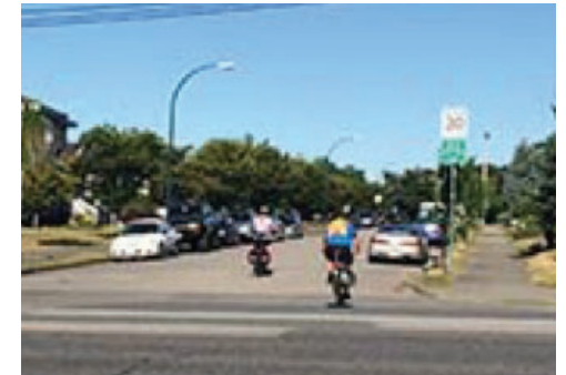
III. SHARED BIKEWAY (Beacon Avenue) Bicycles and vehicles share the lane in a single-file manner. Signage identifies the route as shared and "sharrow" (or other) paint markings indicate the intended path of bicycle travel. Vehicle speeds are slowed through intentional street design so that cyclists can maintain speeds similar to vehicles.
