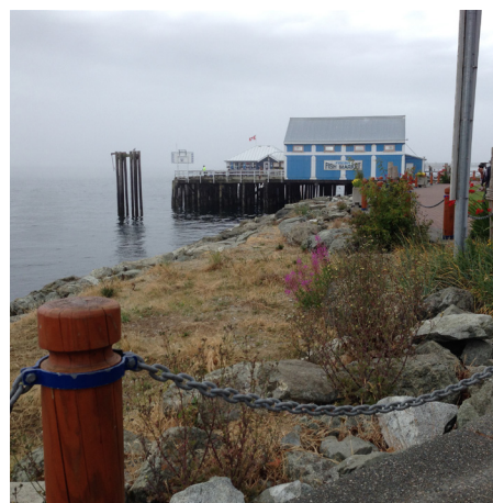
Top of rip rap with Beacon Wharf in background.
