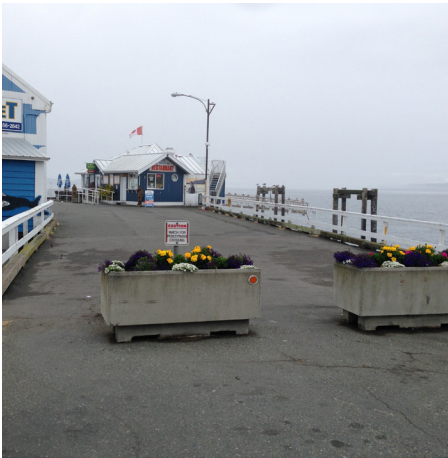
Temporary barriers with pedestrianized wharf area beyond.
