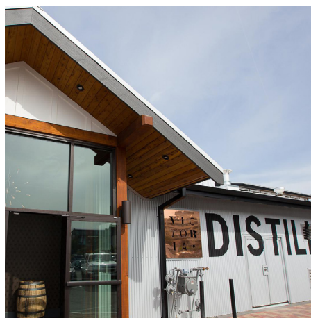
Employ a complementary industrial aesthetic to new waterfront buildings
