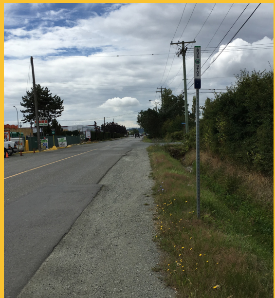
An example of a stop in the West Side with an identification sign but no landing bay nor accessible routes to/from the stop.
