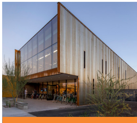
Modern light industrial building with weathering steel
