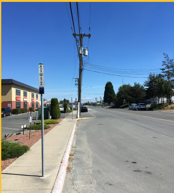
An example of a basic bus stop in the West Side with identification markings, landing bay, and accessible routes to/from the stop.
