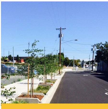
Stormwater swales within a landscaped buffers on an industrial street
