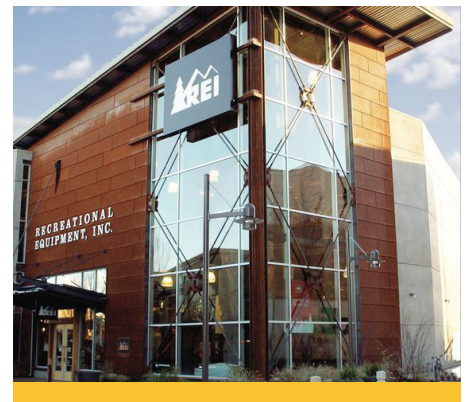
Building architecture with shed roof and industrial aesthetic
