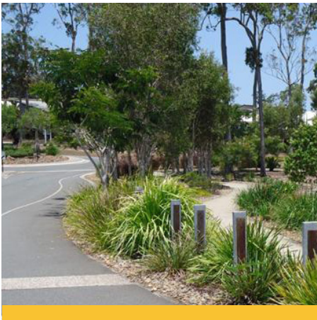
At-grade crushed stone pathway separate from roadway by landscaping
