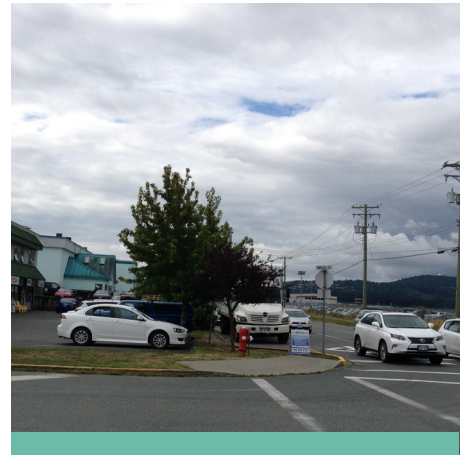
A curb-cut with no sidewalk connections shows the lack of pedestrian amenities and accessibility on the West Side.
