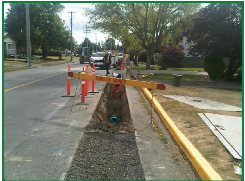
Water main construction
