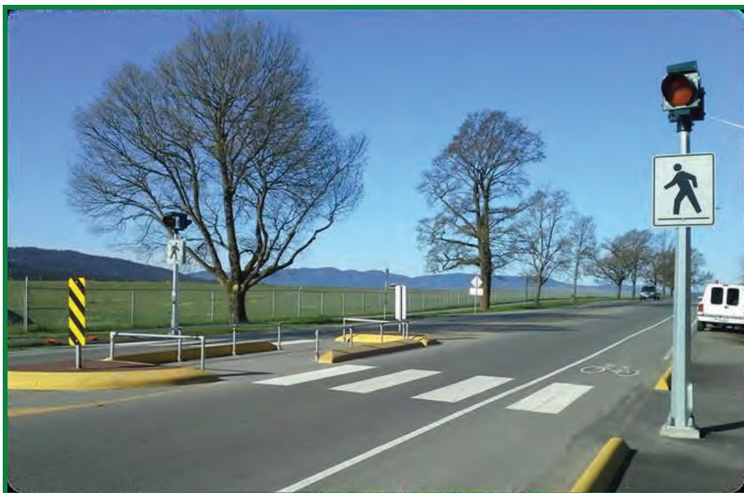
New Crosswalk with pedestrian activated flashing lights on Beacon Avenue West
