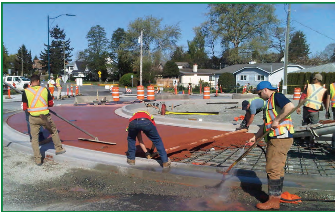
Pouring concrete at the Fifth Street and Ocean Avenue roundabout
