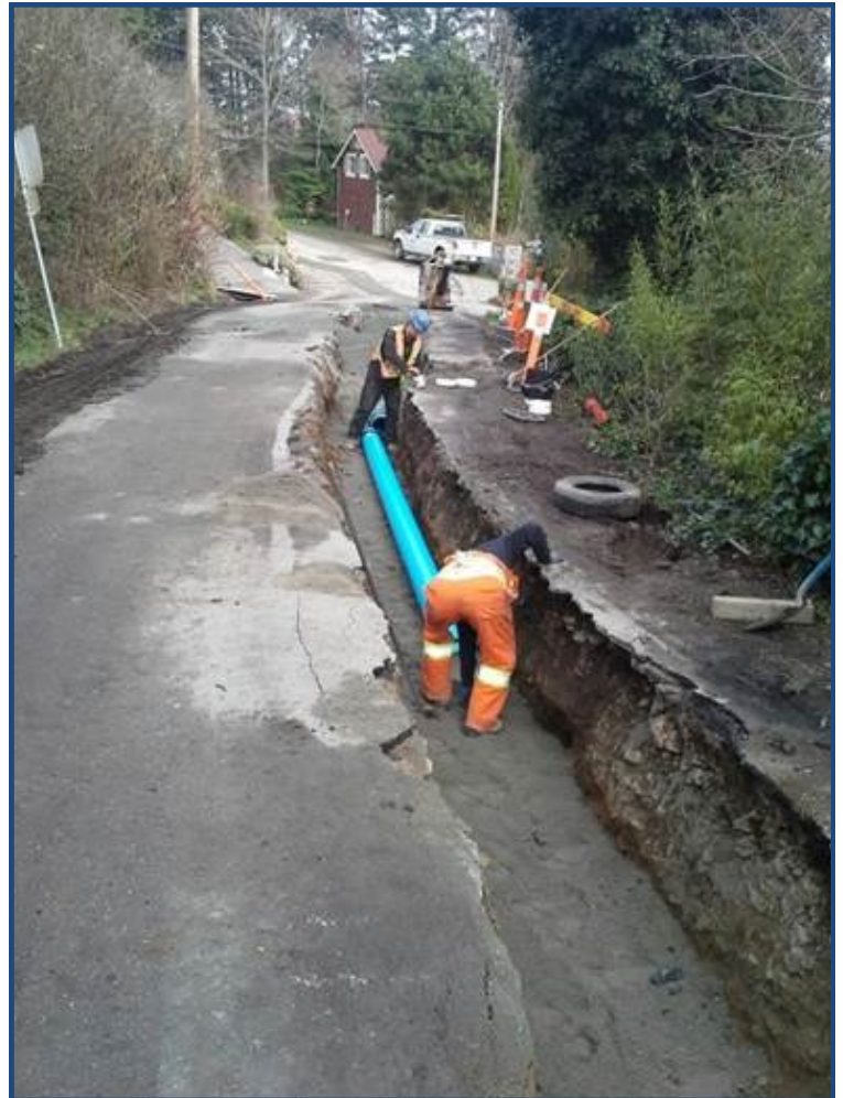
Water main construction on Allbay Road
