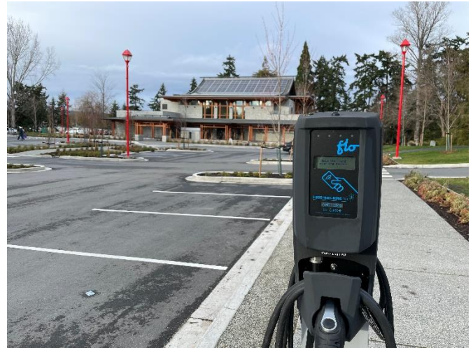
This FLO Level 2 charging station at the Esquimalt Gorge Pavilion in Esquimalt is an example of a “networked charging station”.
